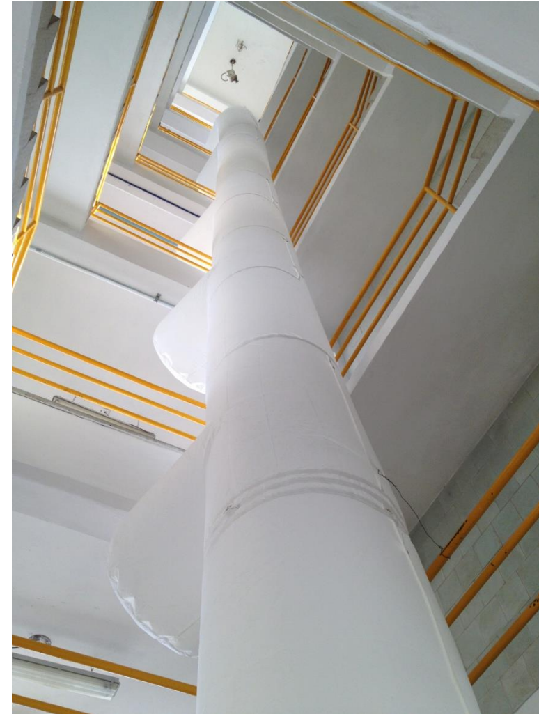
High temperature duct through the 'well' of Stairwell to six floors of the mill
