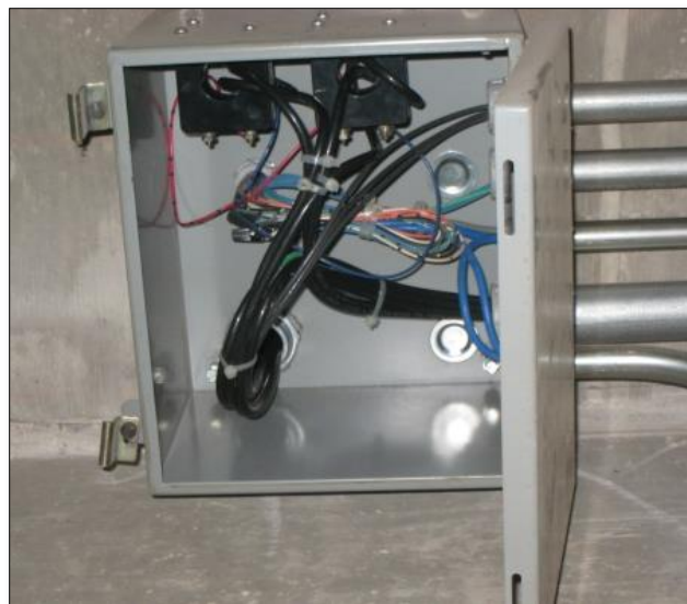
Overhead electrical junction box
